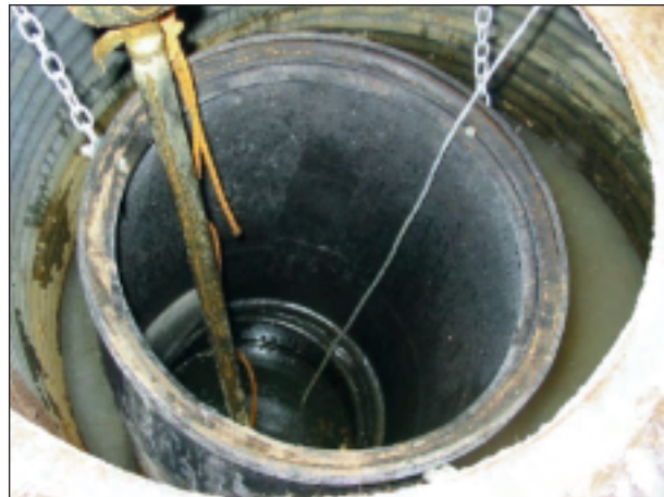
A view of the inside of the wet well showing the arrangement of the plastic drums
