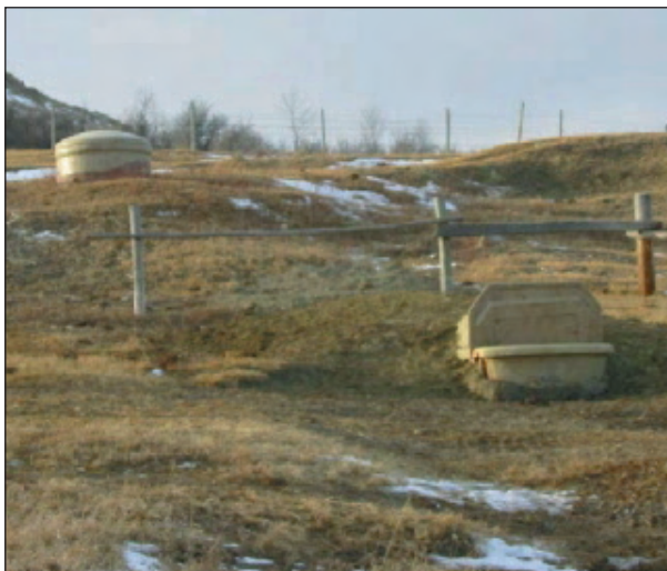
A view of the well and a nearby fiberglass all season water trough, partially buried
