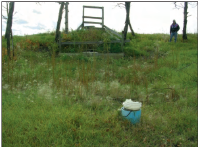
Culvert in bank
