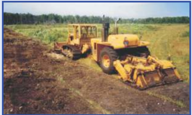
Rotovating harvested site.
