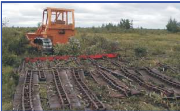
Mechanical – Bulldozer drag used to bark scrape aspen suckers every 2 to 4 years. Photo: Ron Moss
